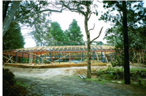
New Dhamma Hall Construction
